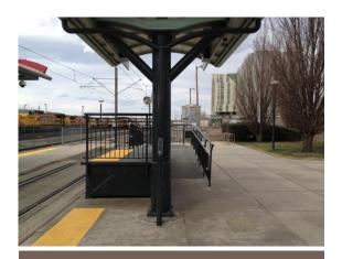
New modular ramps being used at RTD stations
